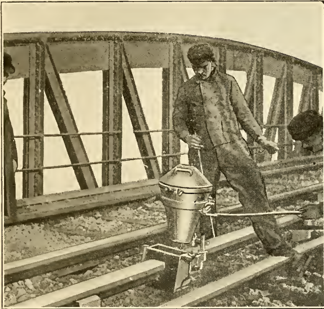
FIG. 70.—Appliances in Position for Welding Third Rail.
